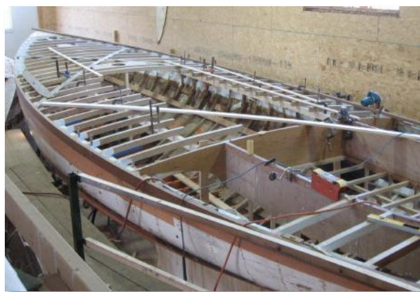
Figure 16 - Deck Beam Construction. (Courtesy Doug Hylan).
