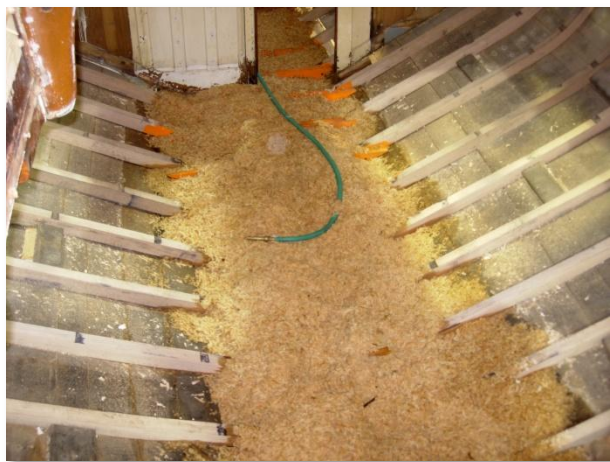
Figure 13 - Frames Replaced. (Courtesy Maynard Bray).
