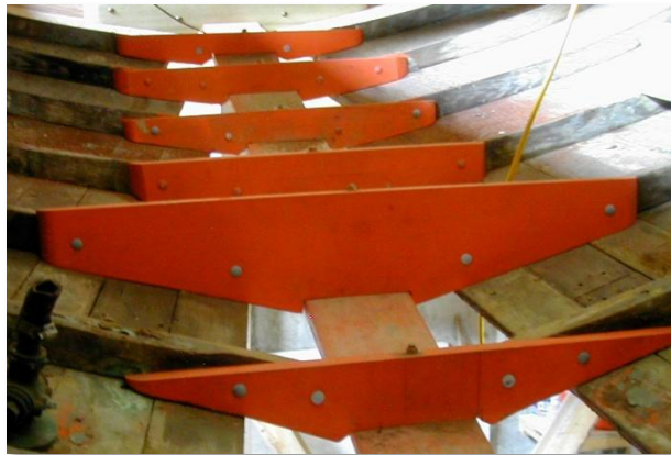
Figure 12 - New Floor Timbers. (Courtesy Maynard Bray).
