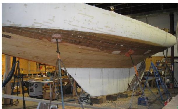
Figure 25 - Planking Complete. (Courtesy Wayne George).
