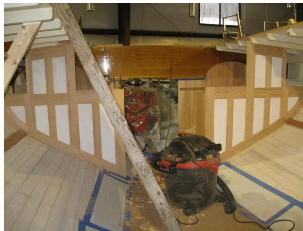
Figure 26 - Early Bulkhead Installation. (Courtesy Wayne George).
